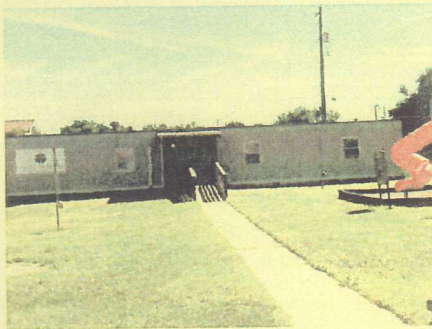
The Johnson Building
