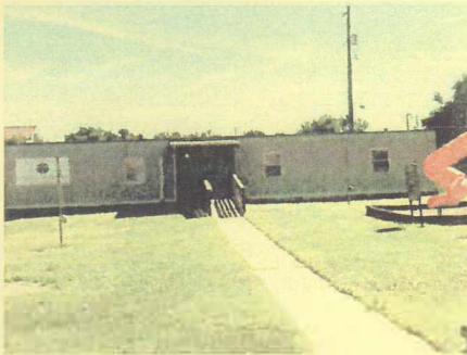
The Johnson Building
